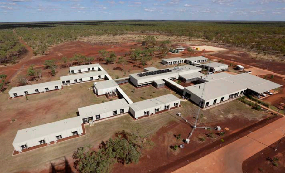
The new facilities at Delamere Air Weapons Range. Defence images.
