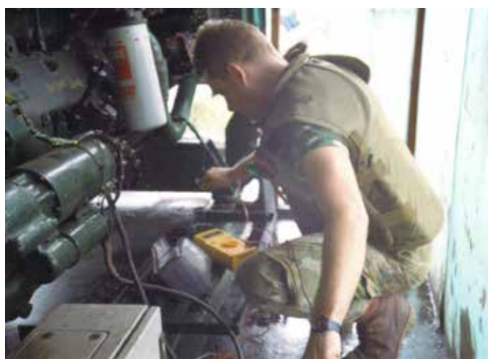
Repairing the Pteah Australii Base Camp Power Generator, Phnom Penh, Cambodia, 1993.
