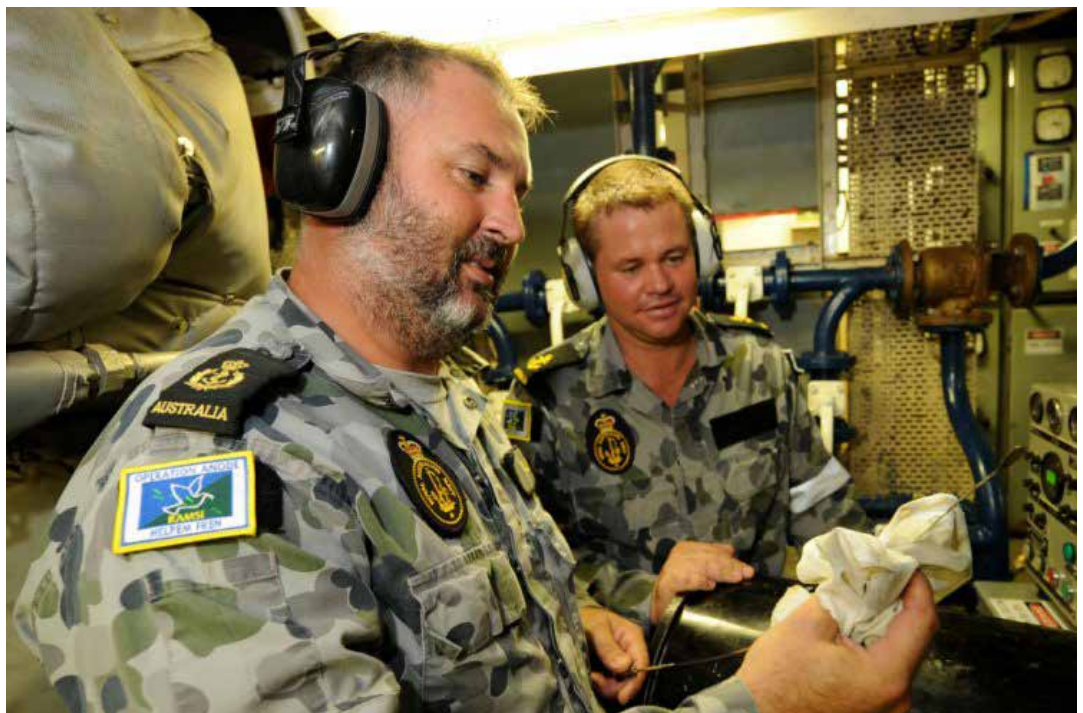
Chief Marine Technician Mathew Philp and Leading Seaman Michael Wilson check the oil in the engine room on HMAS Brunei during operations in the Solomon Islands in support of Operation ANODE - the Australian Defence Force (ADF) contribution to the Australian-led Regional Assistance Mission to the Solomon Islands (RAMSI).
