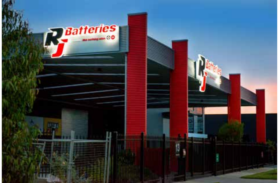
The fascia of R&J Batteries' Truganina, Victoria branch.
