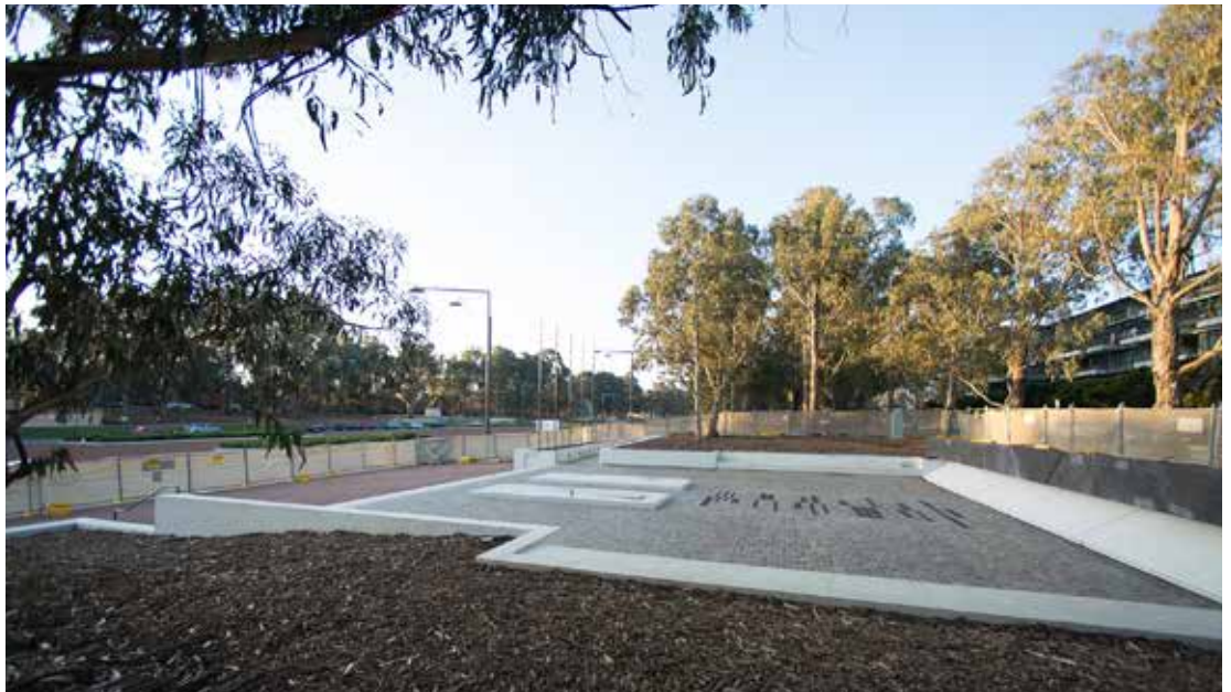
Construction site June 2017
