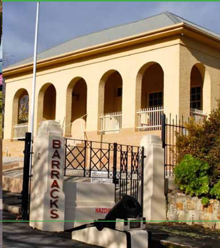
(below) Front gate and guard house at Anglesea Barracks in Hobart
